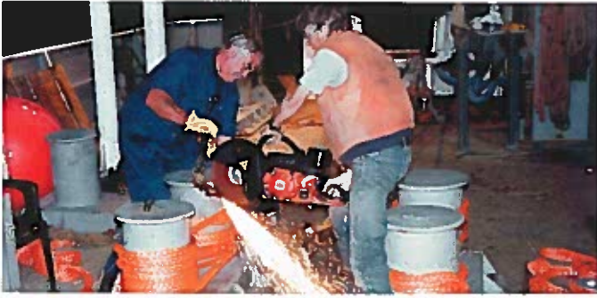
Beecher Wooding (right) and John Hutchings of Margus Undersea Cable Systems cut the cable for splicing into the junction box.
