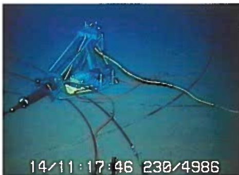
After a cable snapped and unexpectedly sent the termination frame plunging to the ocean bottom, scientists were relieved to find it sitting upright and ready to be plugged in.
