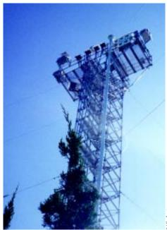
The WHOI aerosol sampler is positioned on the right wing of the 22-meter (73-foot) Bermuda tower. The five filter modules (in a three/two stack) are mounted on the railing to the right.
