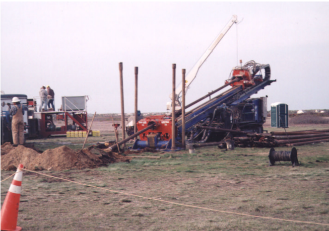
Figure 4: Directional Drilling of Cableway
