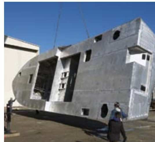
Rollover of the new 60-foot coastal research vessel Tioga in November. The new vessel arrived at WHOI in April 2004, and replaces the 24-year-old Asterias.
