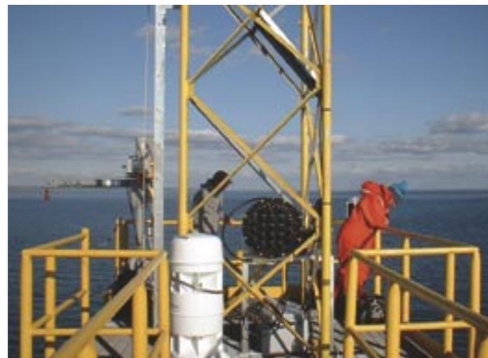
Jay Sisson, left, and Mike Purcell complete connection of the Martha's Vineyard Coastal Observatory Air-Sea Interaction Tower data node (black cylinder at center) with the observatory laboratory ashore. The connection facilitates transmission of a variety of data from tower sensors both above and below the sea surface. The south shore of Martha's Vineyard is in the background.
