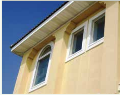
Figure 4-14. Flat impact polycarbonate panels are installed directly over windows of a coastal home. This window covering provides excellent storm protection with minimal aesthetic impact. Image courtesy of Roll-a-way.
