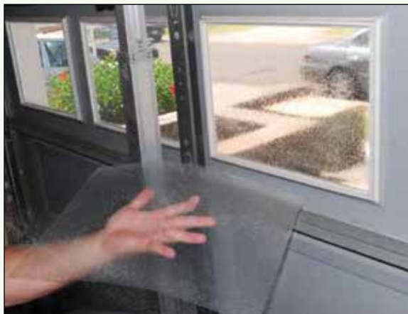
Fig 4-21. Laminated film comes in various thicknesses and strengths. Here the film is applied to an existing window before it is fastened to the frame with silicone structural sealant.
