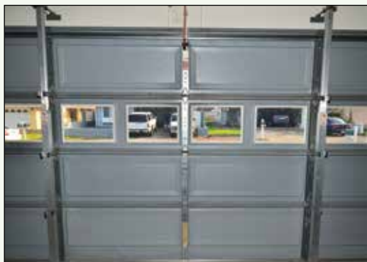
Figure 4-23. Vertical braces such as these can be deployed during high-wind events to strengthen the garage door. The braces are secured from the header over the garage door to the fasteners installed in the concrete floor. Deployment and breakdown are about 10 minutes each. The windows have been covered with a laminate film. Image courtesy of Dennis Hwang.
