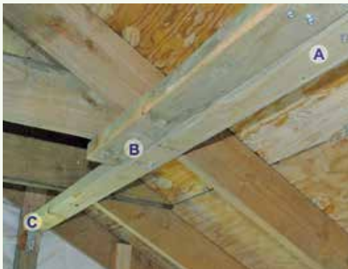
Figure 4-3. In this application of lateral bracing, the 2"x4"s are 18 inches from the ridge and connect to horizontal members that attach the opposing trusses. Not all roofs will have the horizontal members. The 2"x4"s are connected with two #14 3-inch screws (A) and overlap over two trusses (A and B). The end is connected to the gable end with an angle or L bracket (C). Image courtesy of Dennis Hwang.
