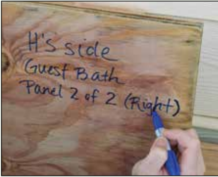
Figures 4-19 and 4-20. Not only is it necessary to install plywood opening covers correctly, it is also important to correctly label them and store them away from heat and humidity. Images courtesy of Dennis Hwang.
