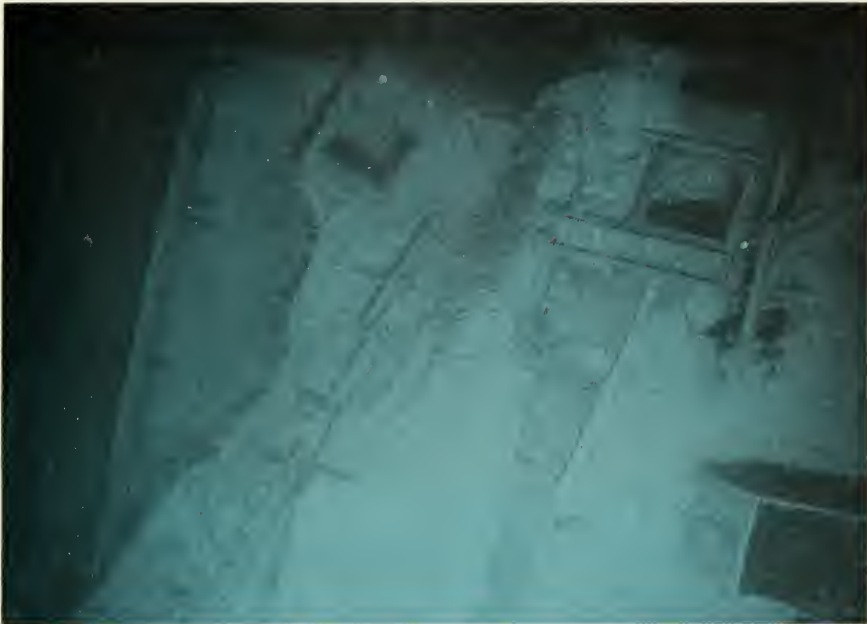
Starboard wing bridge, badly damaged
