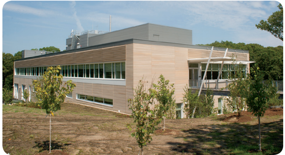
WHOI's newest building: the Laboratory for Ocean Sensors and Observing Systems
