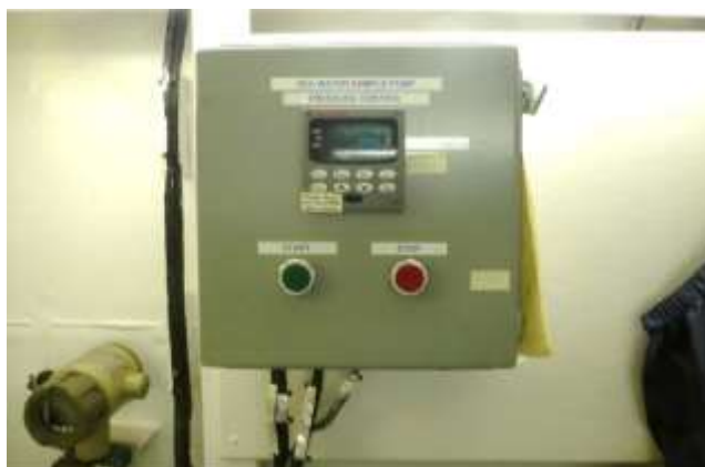
Figure 25. Honeywell controller for the pump, located in the TSG lab.
