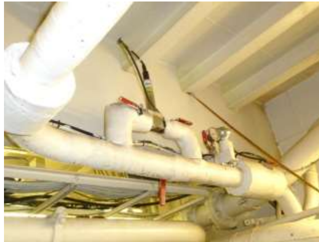
Figure 26. SBE38 temperature sensor in the engine room. This picture is from a previous year and during the winter refit 2016-2017 changes were made to the plumbing but essentially this is the same configuration.
