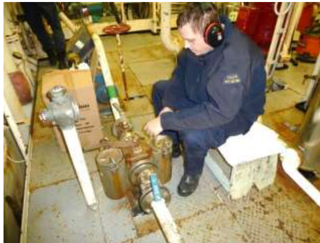
Figure 24. Seawater passes through a filter before going to the pump (in background). When the ship is in sea-ice the flow is switched from one filter to the other to allow the necessary frequent clearing out of slush from the filter. This picture is from a previous year but is the same strainer configuration for 2018.
