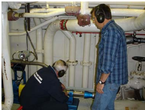
Figure 14. Pump for seawater loop at intake in engine room.
