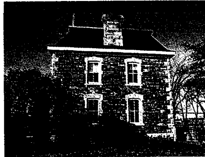
PHOTO 128: Distinctive red sandstone of the Jacobsville Group, quarried during excavation of the locks, was used to construct the buildings at Sault Canal National Historic Site.
