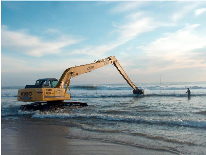
**Figure 1.** Backhoe excavating a hole in the inner surf zone near Duck, NC, at low tide.
