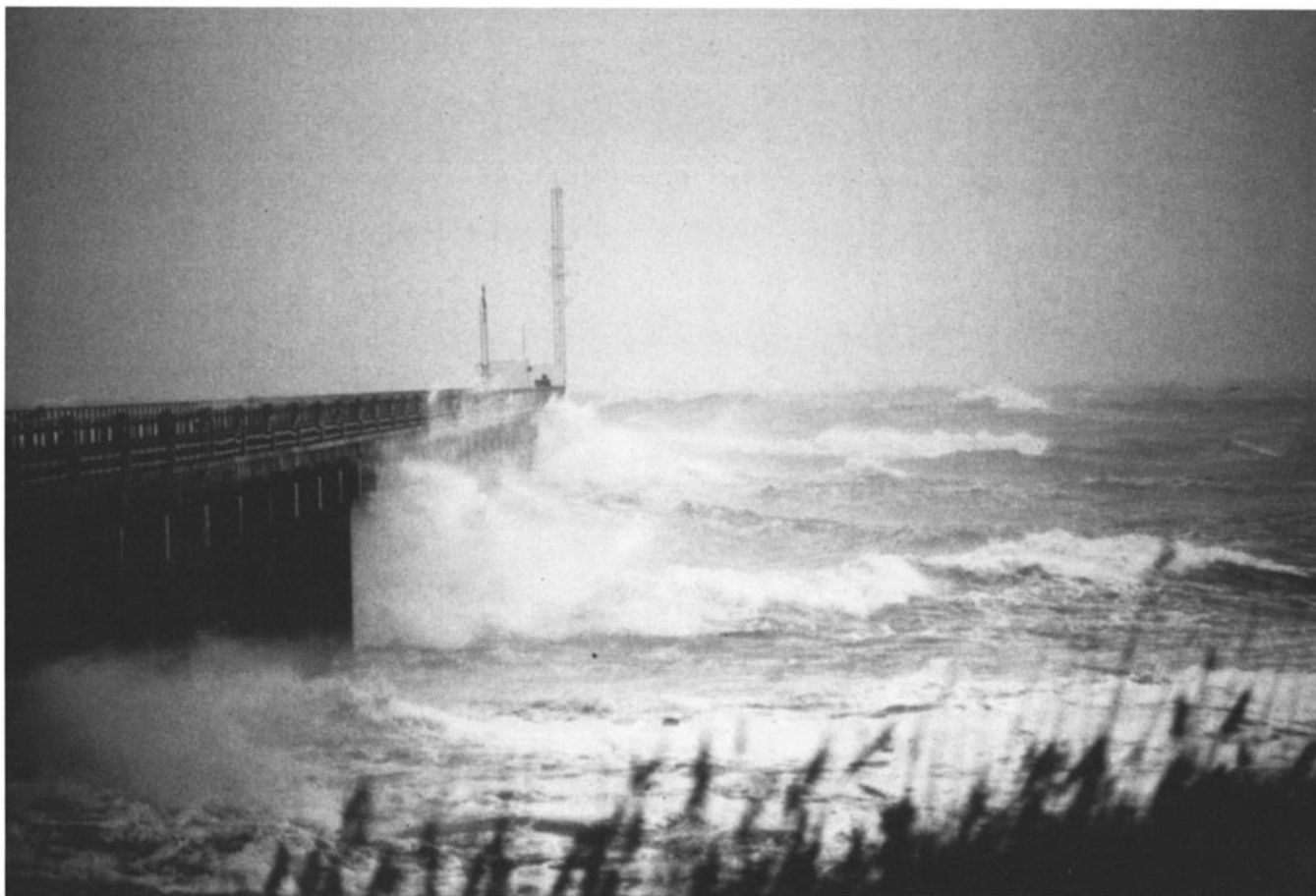
Figure 1. Photograph showing two breaking waves (in about 2 and 5 m depths) at the U.S. Army Corps of Engineers' Field Research Facility pier (the deck is about 7.5 m above mean sea level). The surf zone extends more than 1 km offshore. The gages in 8 and 13 m depths are located about 0.2 and 1.2 km offshore from the pier end, respectively.
