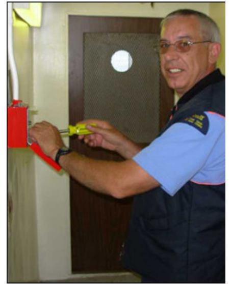
Electrical Officer Stephen Colp services a faulty alarm box.
