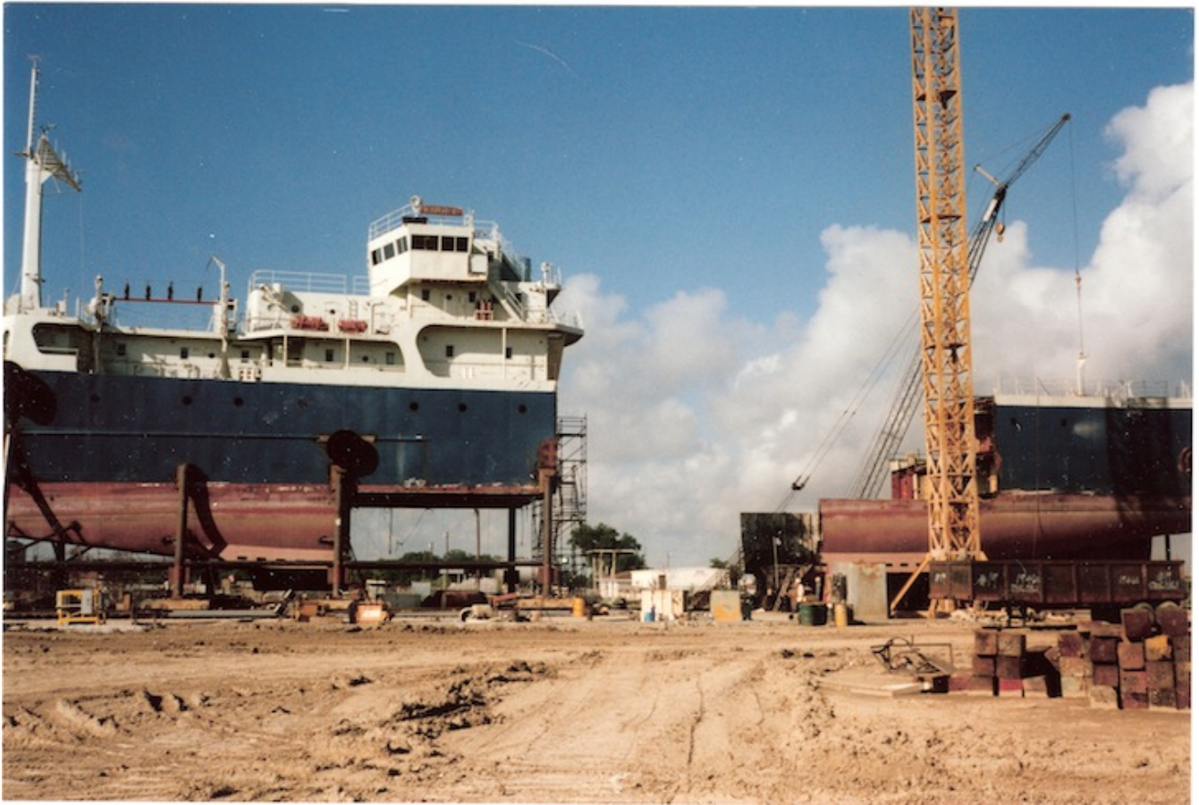
You can see the two halves of the Knorr, gutted and separated, awaiting the arrival of the new section. (Credit: Wayne Sylvia)
