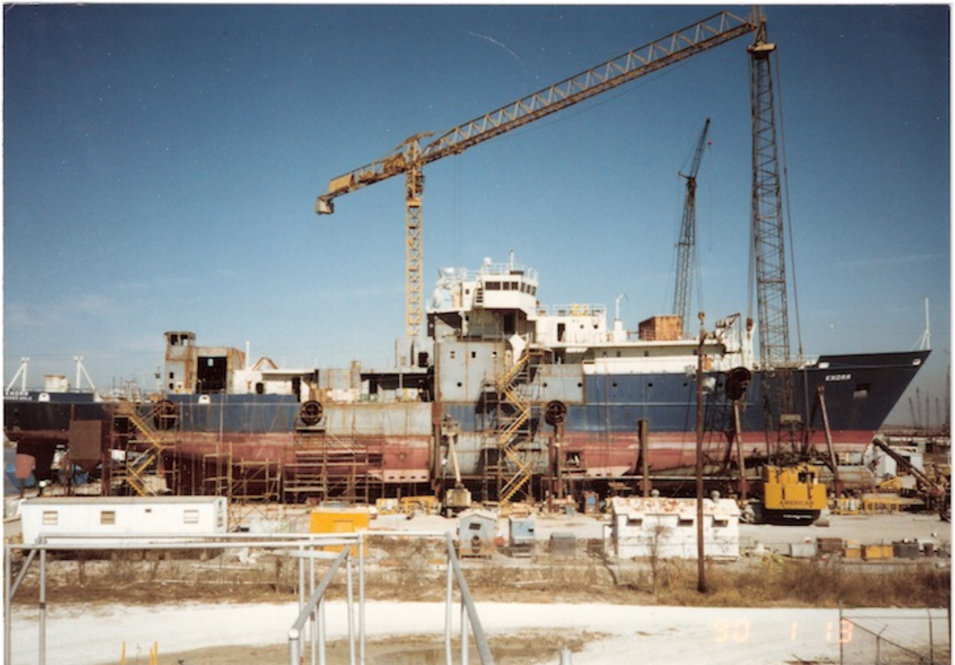
QS8_05d.JPG The Knorr's new section has been welded to the original bow and stern. What's blue and red is the "old" Knorr, what's gray is the new section. (Credit: Wayne Sylvia)
