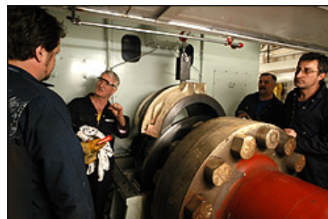
From left, David Walsh, Stephen Hewens, Larry Colbert, and Jim Gale prepare to reassemble the half-ton shaft bearing.
