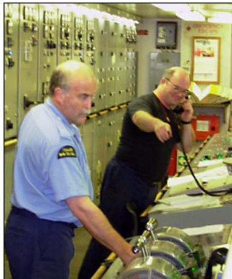
The control room is the heart of the Louis . Here Engine Room Technician Dave Ramsey and First Engineer Michael Willis monitor the Louis ' powerful propulsion system.
