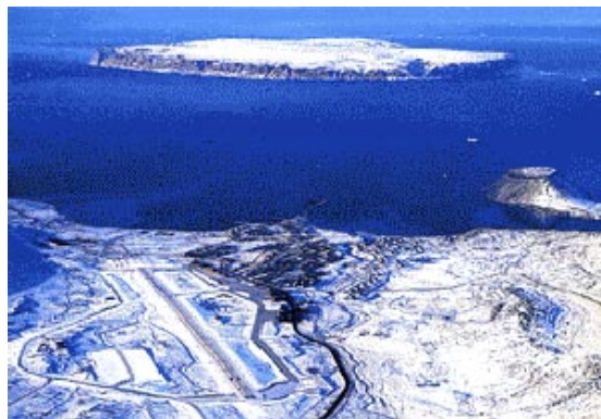
Thule Air Base. (Image courtesy Michael Salling)
