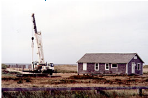
Construction of the meteorological mast next to the Donnelly House.
