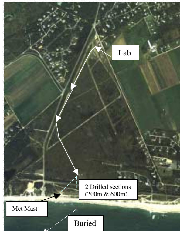
Fig. 1: Aerial View of project site at Katama Air Park showing cable route, lab and met mast sites.
