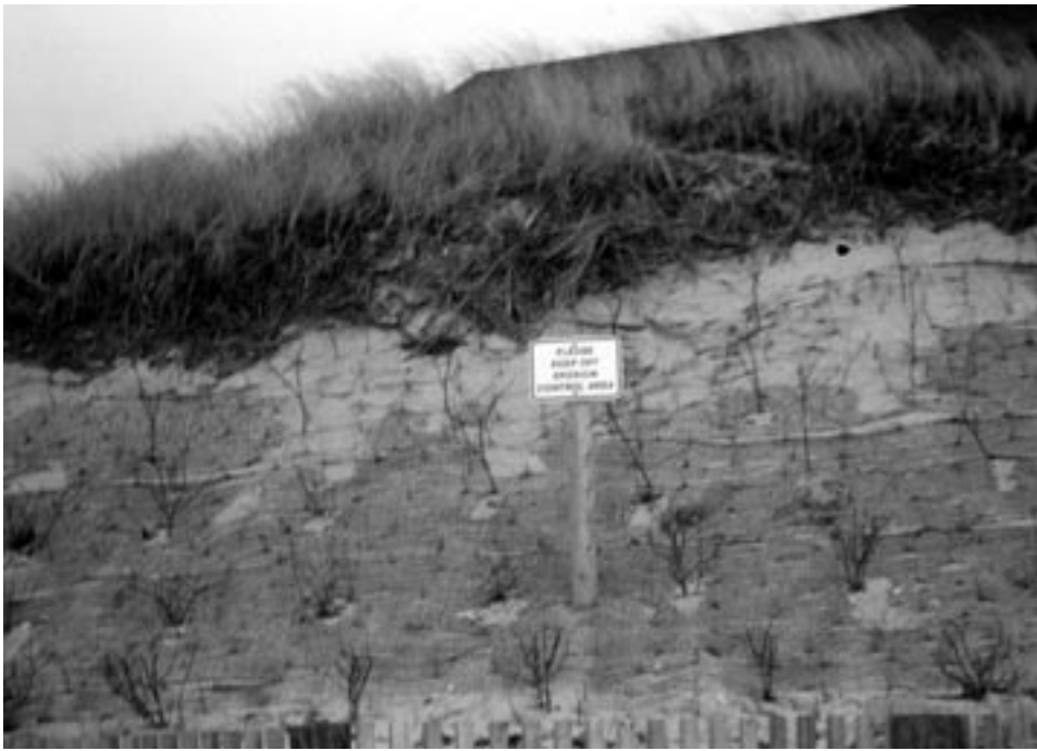
Fig 25. Coastal bank stabilization with a variety of coastal plants
