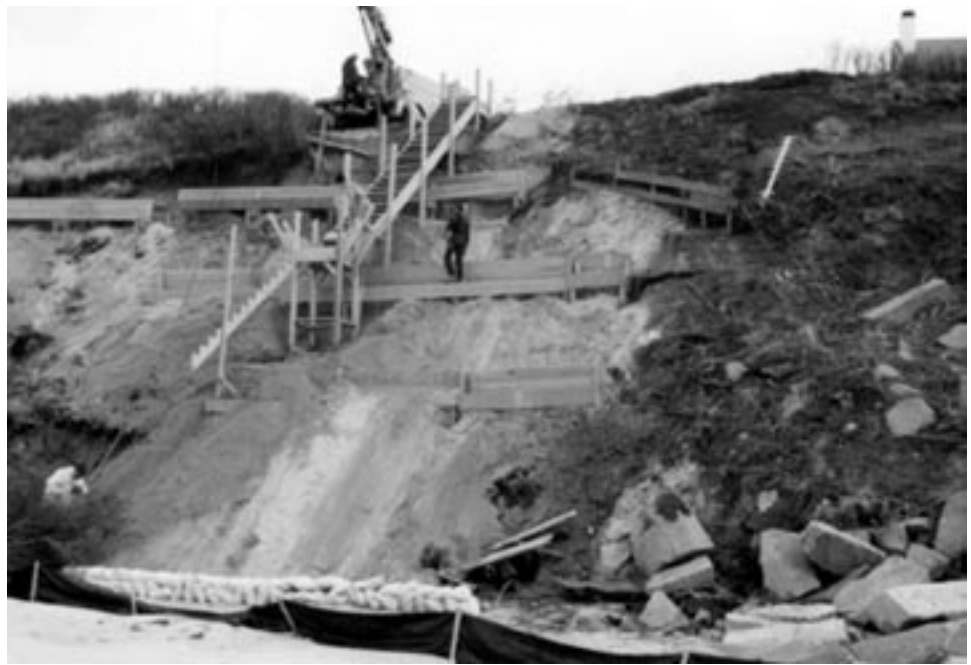
Fig 27. Terraces built across the coastal bank
