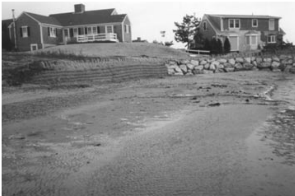
Fig 36. Using fiber rolls to construct a return
