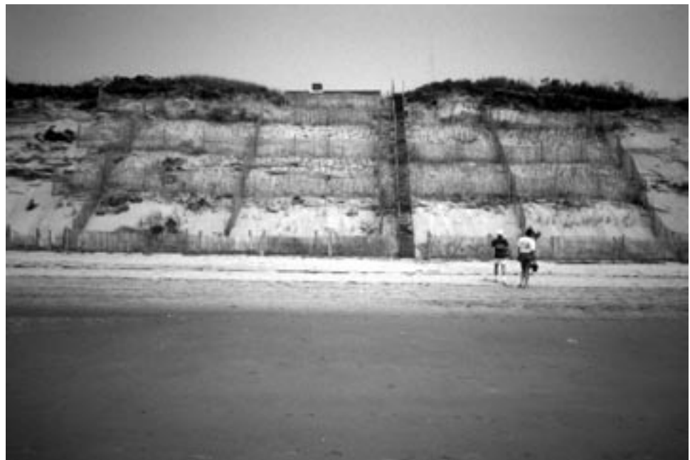
Fig 2. Partially successful non-structural erosion control on a coastal bank
