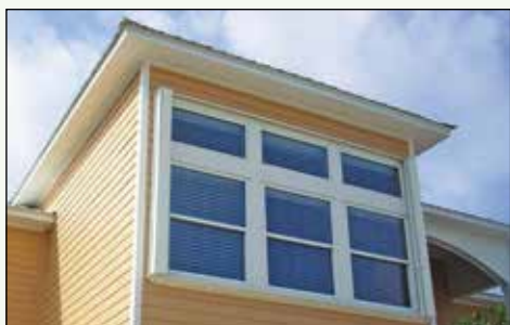
Figure 4-10. Accordion shutter (shown in the open position) installed over a large window of a coastal home. Shutter has been installed to allow deployment from inside the home. Image courtesy of Roll-a-way.
