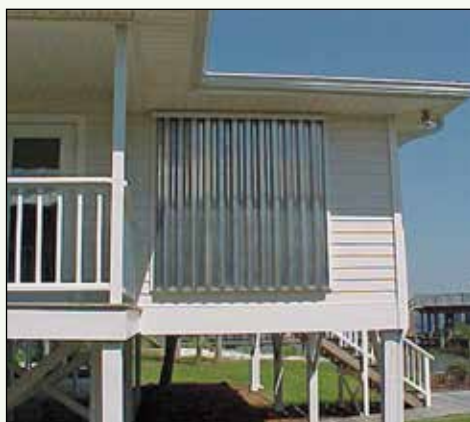
Figure 4-12. These 0.050 gauge aluminum storm panels offer cost effective storm protection. In this example, panels slip into a track above the window and secure onto a bottom track using wing nuts. Image courtesy of Roll-a-way.
