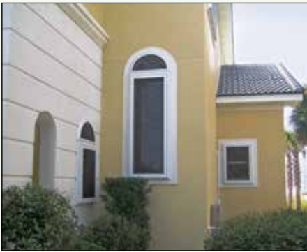
Figure 4-13. In-place stainless steel impact screen protects several windows of a coastal residence. This system requires no deployment and provides shade. Image courtesy of Roll-a-way.
