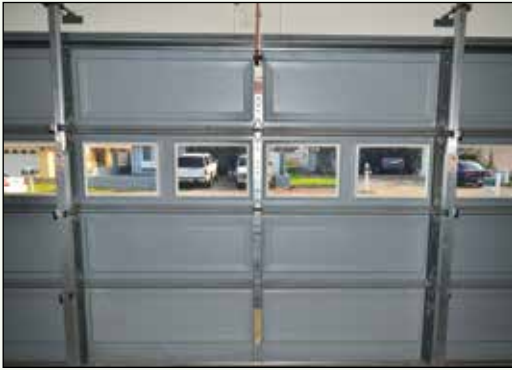
Figure 4-23. Vertical braces such as these can be deployed during high-wind events to strengthen the garage door. The braces are secured from the header over the garage door to the fasteners installed in the concrete floor. Deployment and breakdown are about 10 minutes each. The windows have been covered with a laminate film. Image courtesy of Dennis Hwang.
