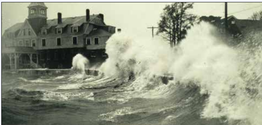
Figure 2-4. The south side of Main Street, Woods Hole, MA during the 1938 Hurricane. Bureau of Commercial Fisheries building on left. Photo Credit: NOAA Photo Library, NOAA Central Library; C&GS Season’s Report Thomas 1938-84.
