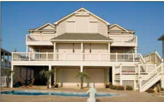
Figure 4-9. Coastal home protected with roll-down shutters on all windows and doors. The shutter is held in place by vertical guide tracks and can be deployed manually or with an integrated electric motor. Image courtesy of QMI, Inc.
