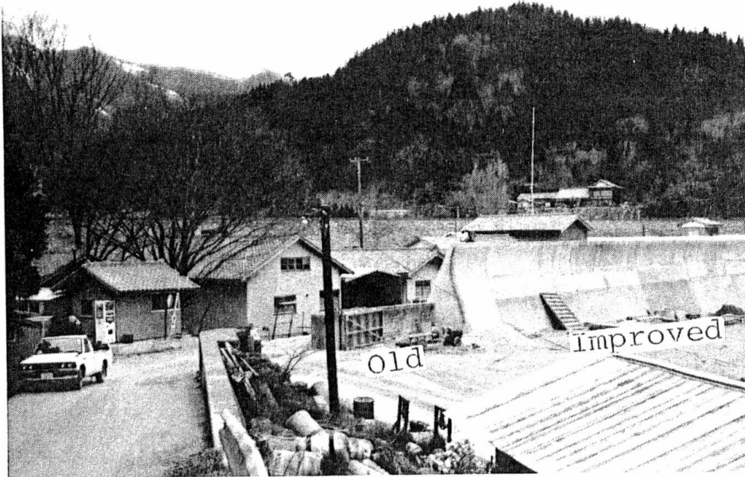
Photo 4. Contrast of old part and improved part of a tsunami wall.
