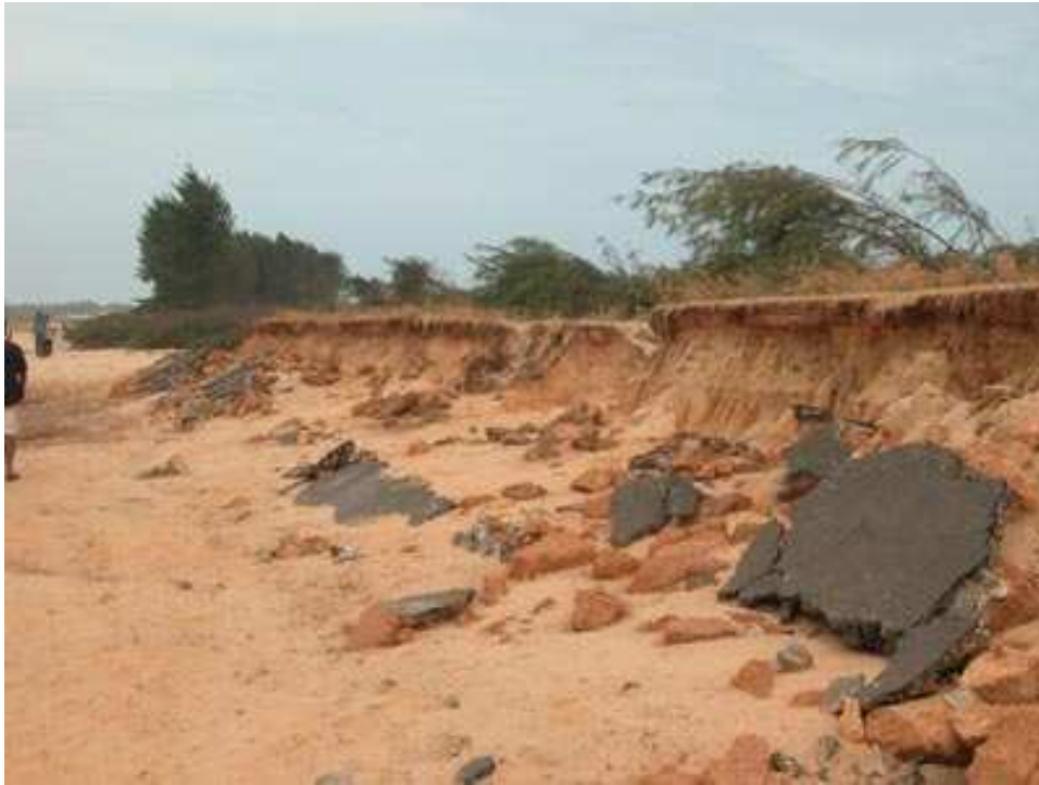
Road bed destroyed at Panadura, Sri Lanka, 26 Dec. 2004
