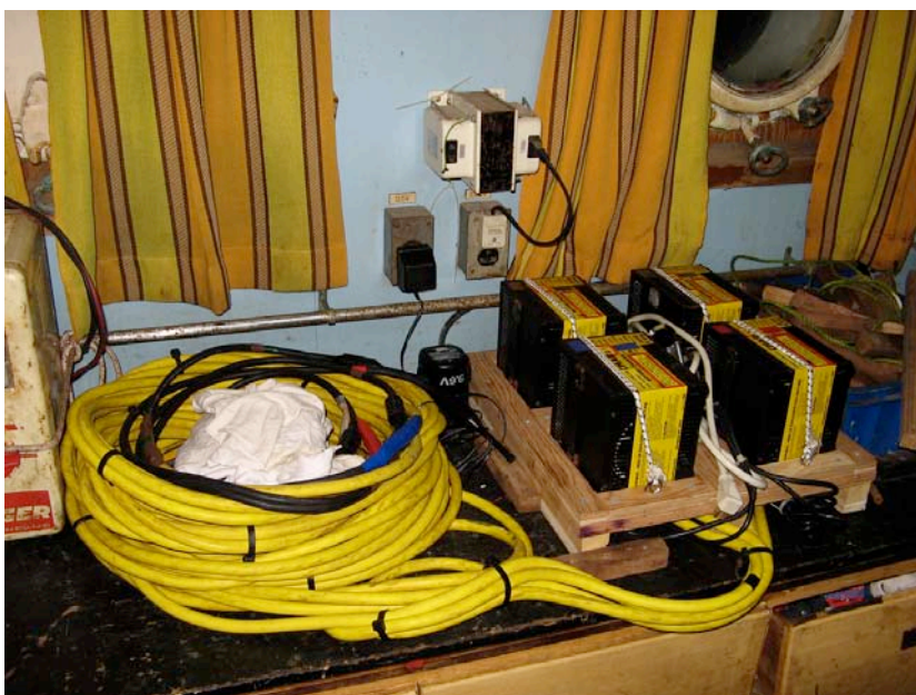
Figure A18. Battery chargers and cables for TowCam DSPL SeaBatteries.
