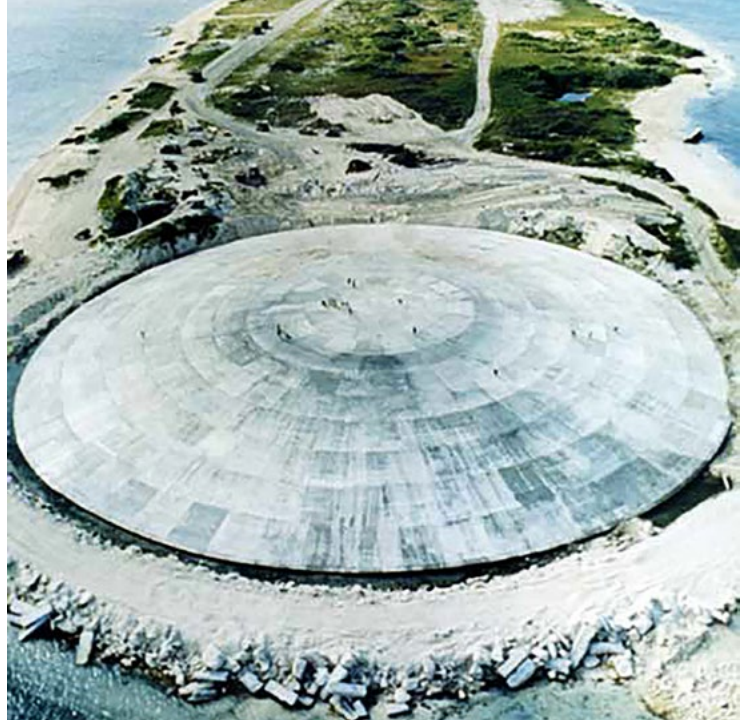
The Runit Dome on Enewetak was constructed in the late 1970s. The United States bulldozed some 11,000 cubic yards of radioactive topsoil and debris into a crater from a nuclear bomb test and then sealed it over with concrete in an attempt to contain radioactivity. Is seawater leaching underneath the Runit Dome and transporting radioactive compounds into the ocean?
