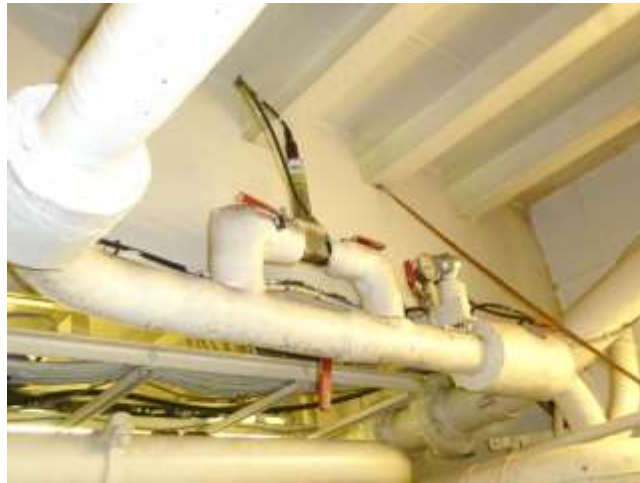
Figure 8. SBE38 temperature sensor in the engine room. This picture is from a previous year and during the winter refit 2016-2017 changes were made to the plumbing but essentially this is the same configuration.
