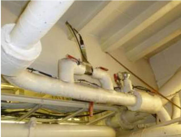
Figure 8. SBE38 temperature sensor in the engine room. Data are brought up to the TSG lab and added into Seasave Acquisition with the lab TSG data.
