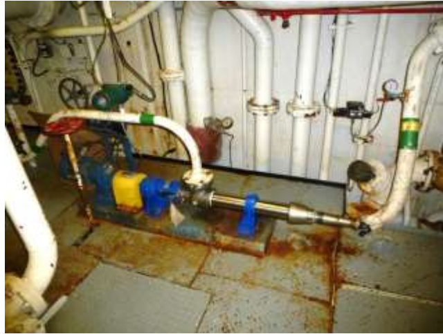
Figure 5. The Moyno pump installed in the engine room.
