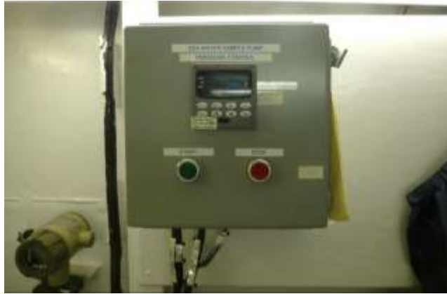
Figure 7. Honeywell controller for the pump. Controller is located in the TSG lab.
